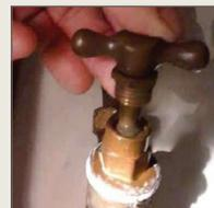
cold water feed with the other end connected to the boiler system. If you find that one end of the metal hose is not connected there may be a cap on the end of the pipe and it will need to be connected to allow water to be injected. To connect, remove the cap from the end of the pipe work and attach the other end of the metal hose. You will then need to tighten this connection with your fingers, **do not** over-tighten with a spanner.
